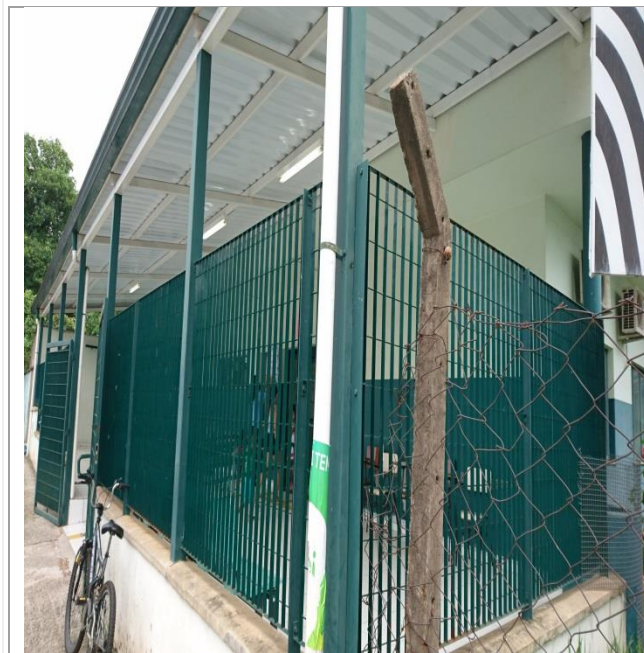
Fachada principal adequada
